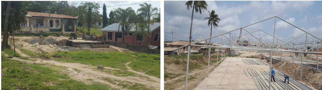
Figure 4: Building structures around the project site
